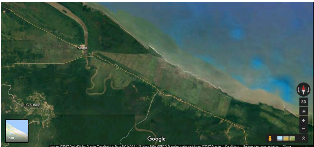
FIGURE 31 : POLDER DE MANA, GUYANE (SOURCE : GOOGLE MAPS)
