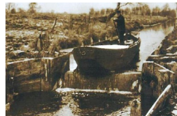
Figure 5b Flap weir (Klappstau) in NW Germany with a fully passable, flexible weir.
